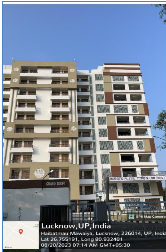
Type-3 Flats in the New Campus
